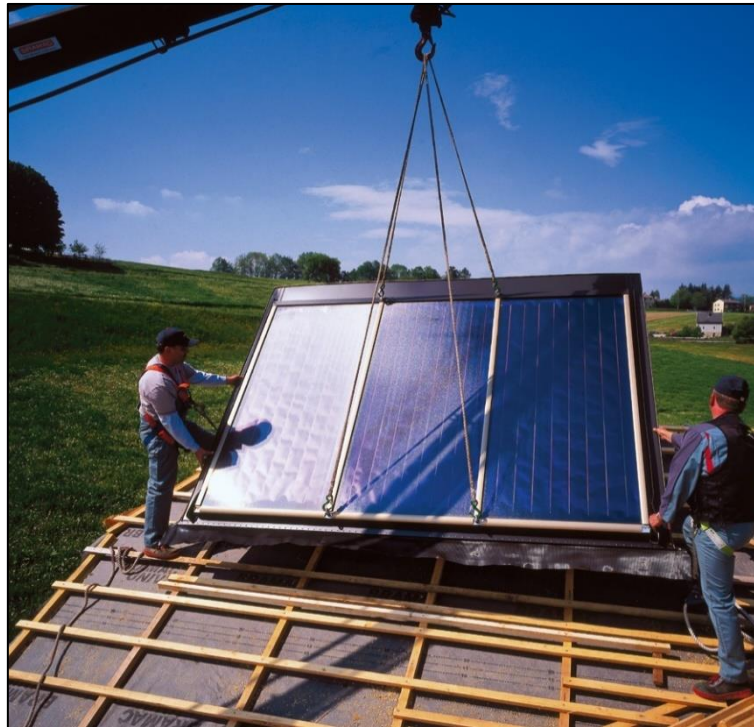
Figure 23. Installing solar thermal collector
