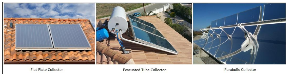
Figure 15. Solar collector types
